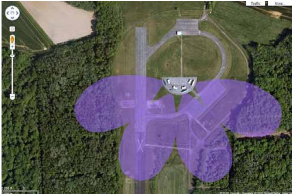
Figure 4.3 Overhead view of the Graves Radar Transmitter
